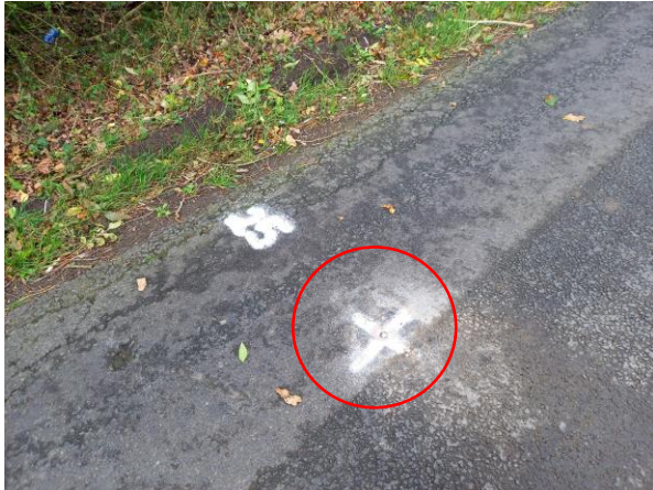
Levelling stud installed hard paved areas
