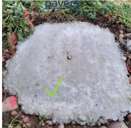
Levelling stud installed soft Ground
